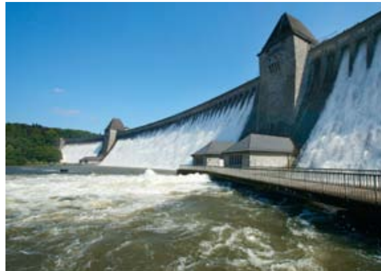
Flood discharge via the spillway of the Möhne Dam in August 2007.
