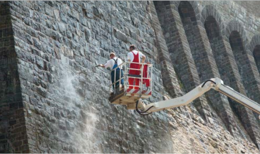
Cleaning walls at the Möhne Reservoir.
