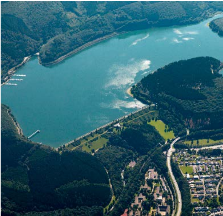
The Bigge Reservoir is one of the Ruhrverband's eight reservoirs.
