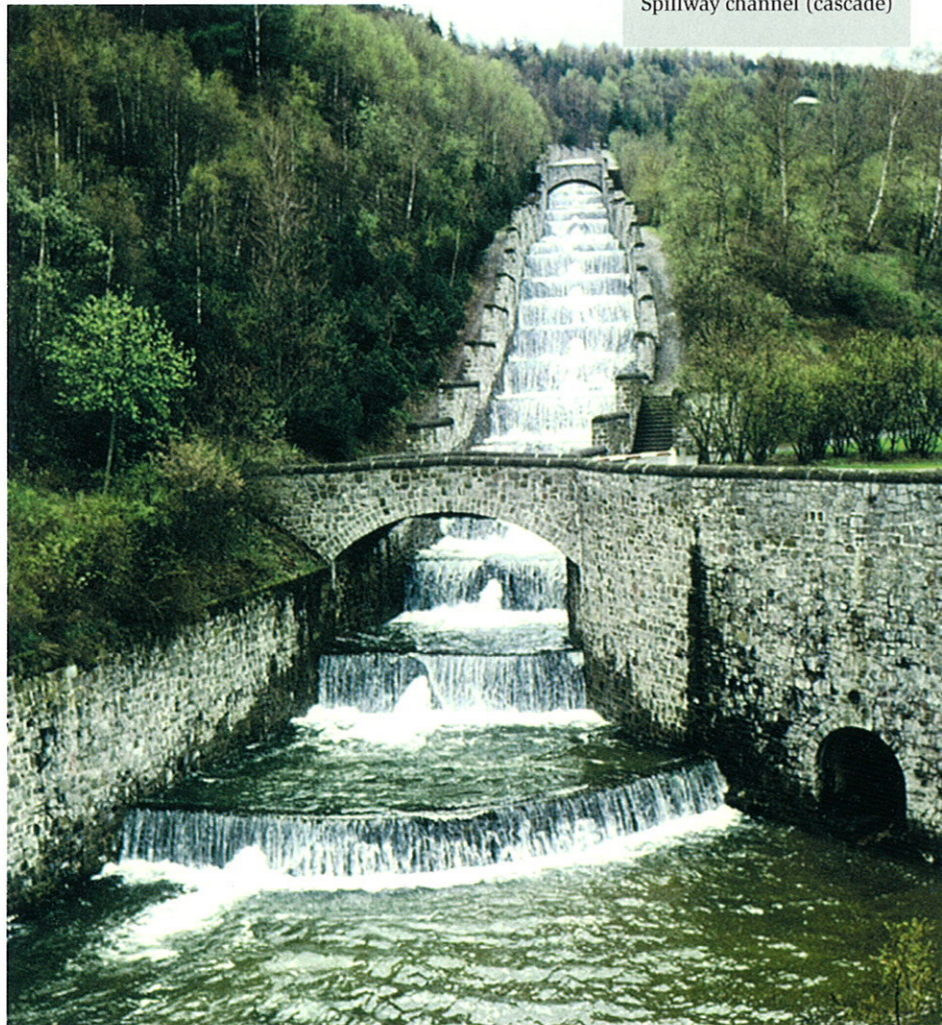
Spillway channel (cascade)
