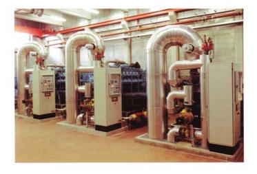
then used for the generation of energy and compressed air in gas motors. The waste heat thus caused is used in turn for providing the digestion tanks with the temperature needed. Additionally, the buildings of the wastewater treatment plant are heated with this waste heat.
