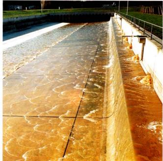
constant level of water of about 1 m. Due to temporalily influx of wastewater the ponds have to be aerated intermediately. Thus, the biological process of decomposition of pollutants is supported and the emission of odour is prevented.
