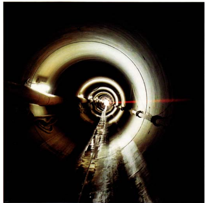
Wastewater tunnel Ludwigstal
